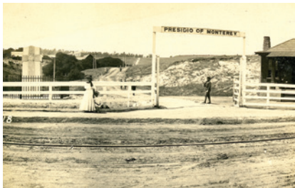
Lower Presidio Gate c1907, courtesy California History Room, Monterey Public Library
