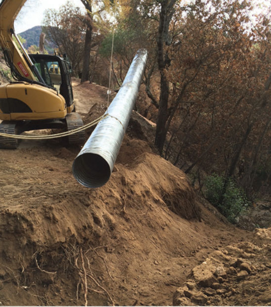
Culvert repair made possible by Soberanes Fire Fund donors
